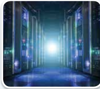
Atlas Control Center Facilities
