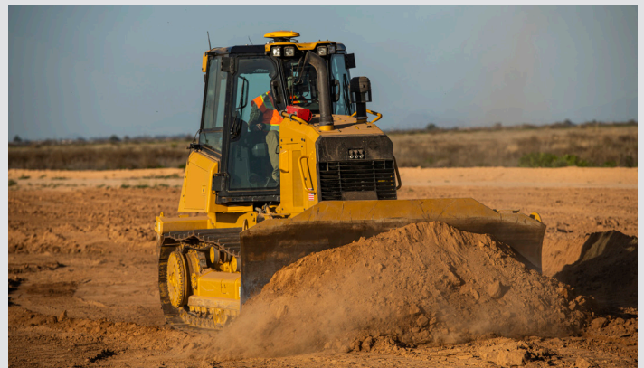
SITE PREPARATION - COARSE GRADING
